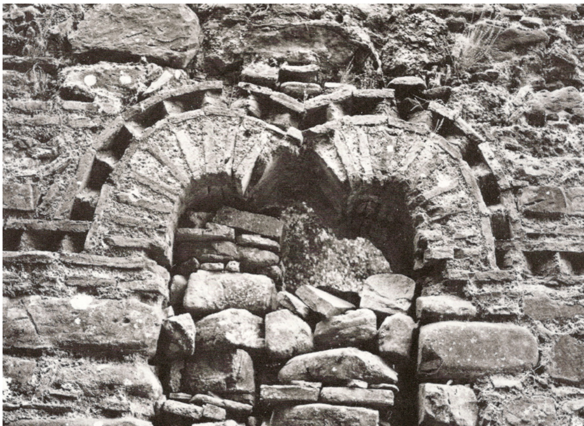
Fig. 47. Mt. Arakynthos, Panagia Trimitou, SW building. Detail of the E façade.
